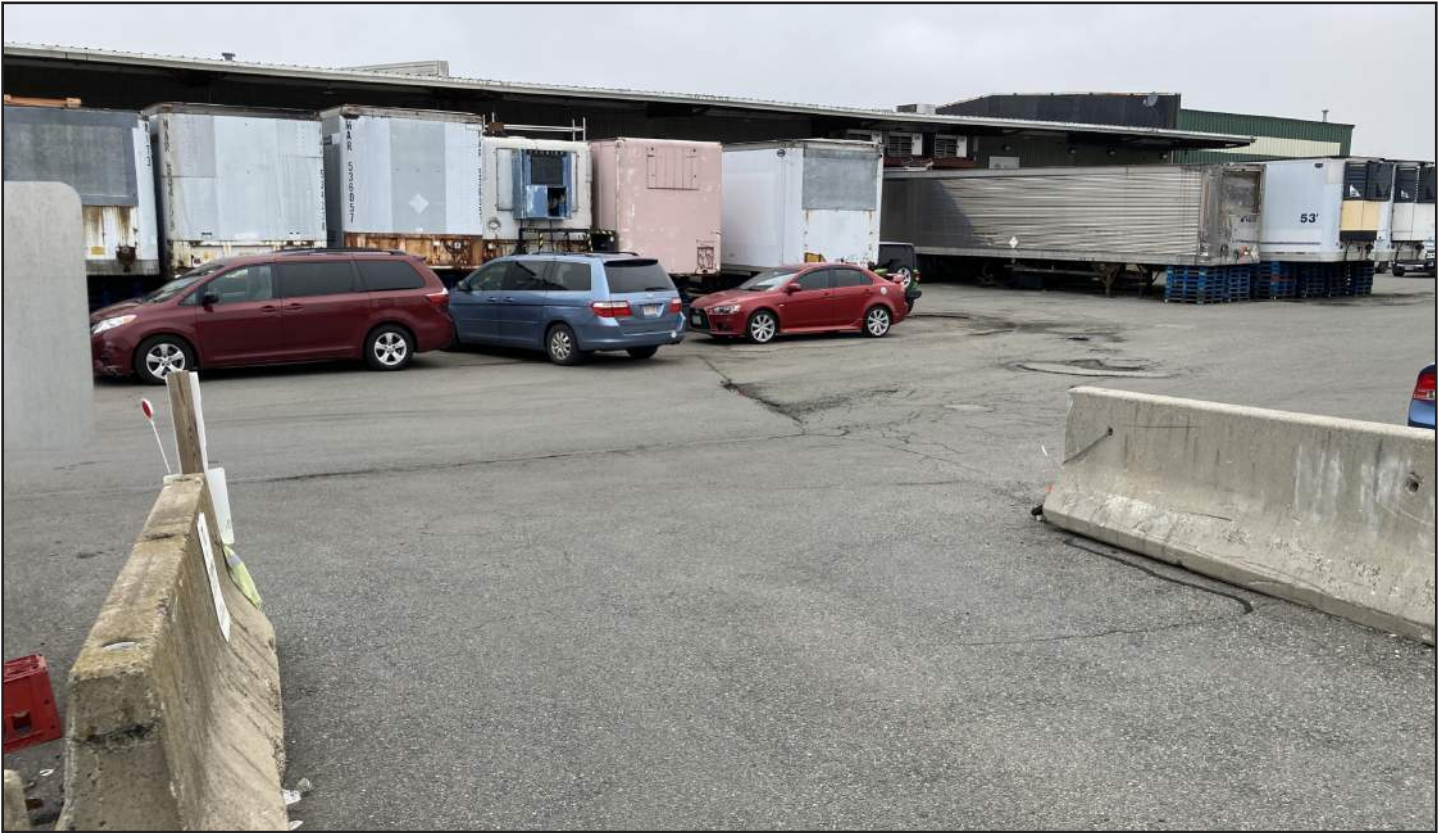
Photograph 5: View of the #155 Market Street facing west along ramp up to dock and upper parking area
