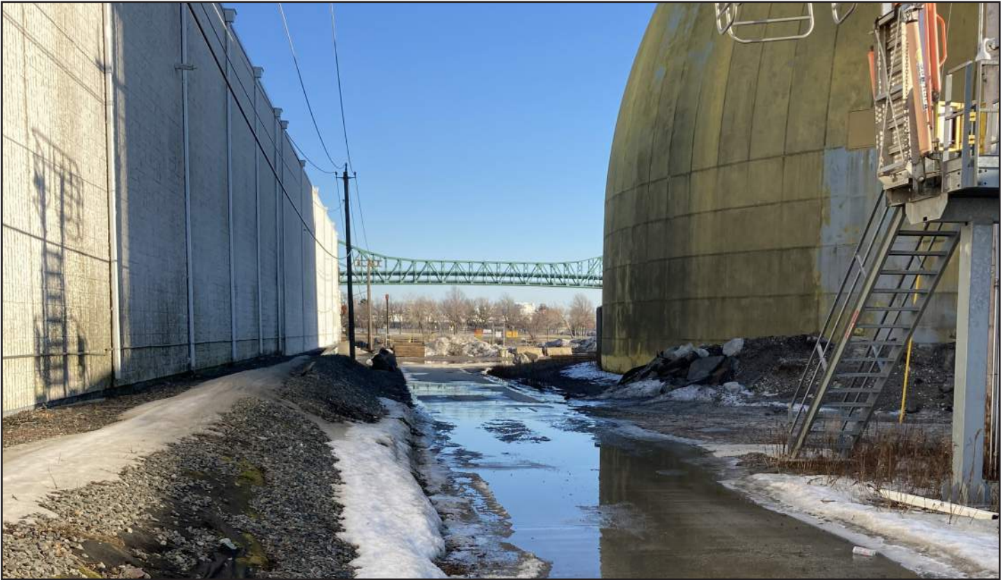
Photograph 13: View looking east towards Island End River, between Lineage Logistics and Quebec Cement
