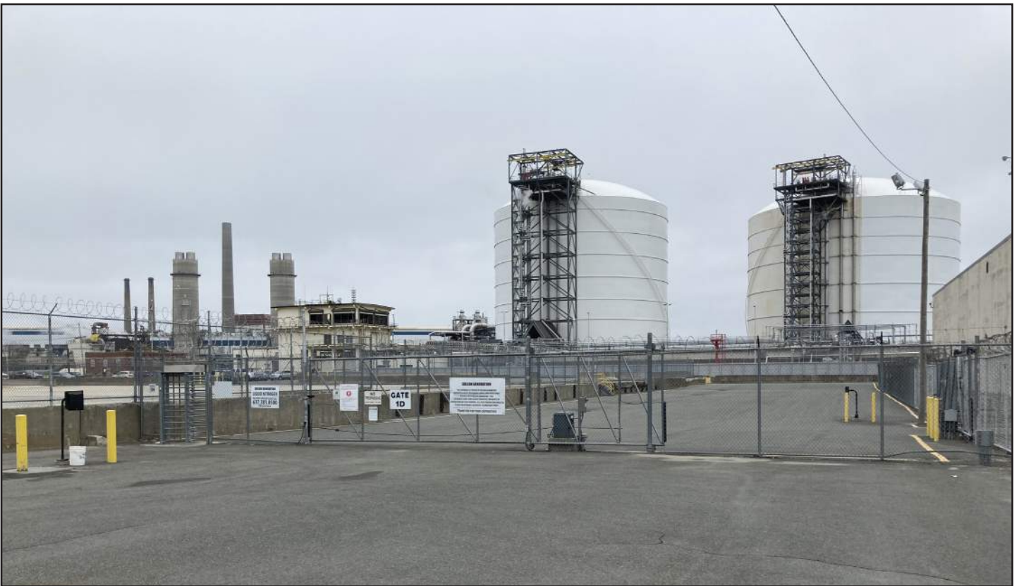
Photograph 14: View looking southwest from Commercial Street towards Constellation Energy
