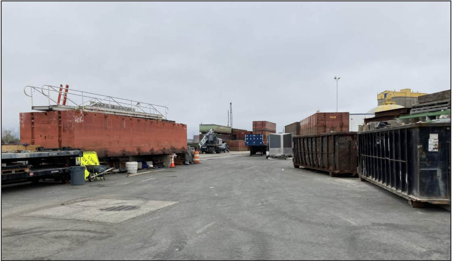
Photograph 9: View of the SPS New England facility facing south towards the southern edge of dock
