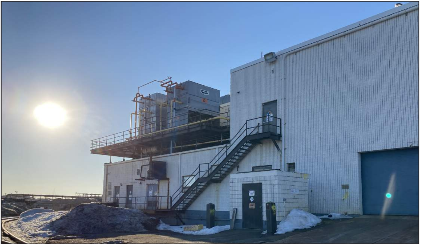
Photograph 11: View looking southwest towards the southeast corner of the Lineage Logistics building
