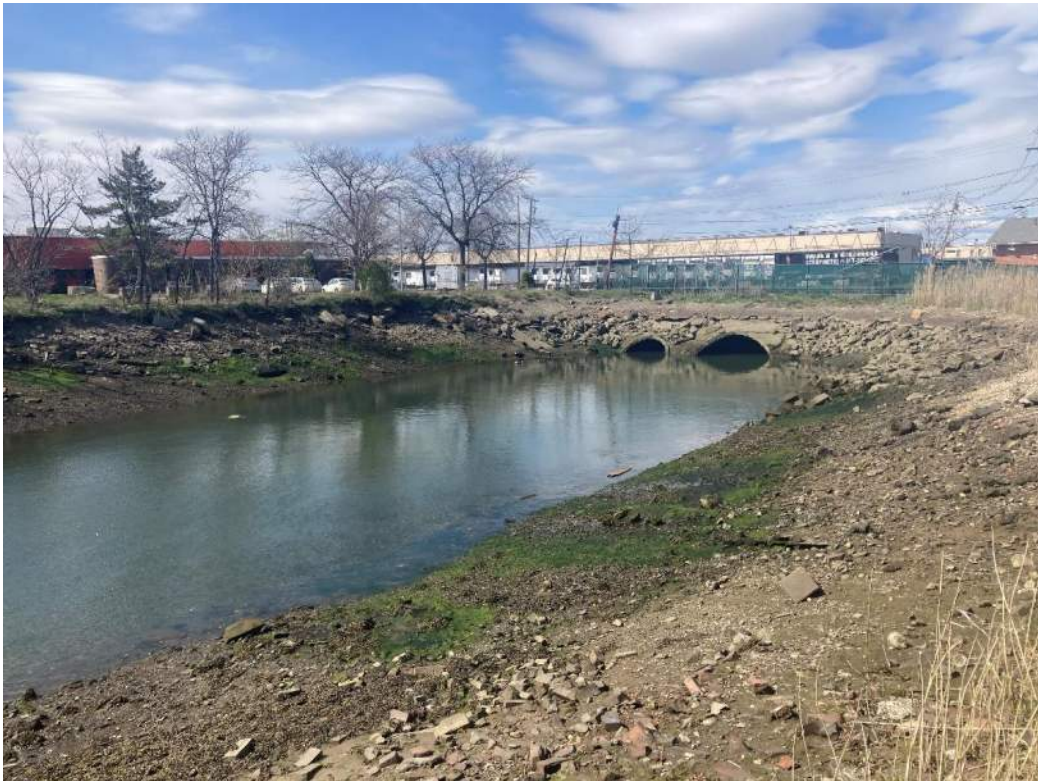
Photo 2: Island End River Culverts
