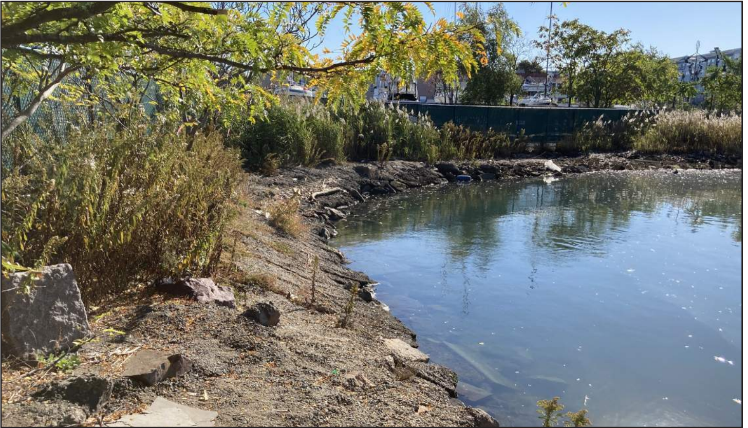
Photograph 1: View of the Island End River behind #359 Beacham Street property and Market Street culvert
