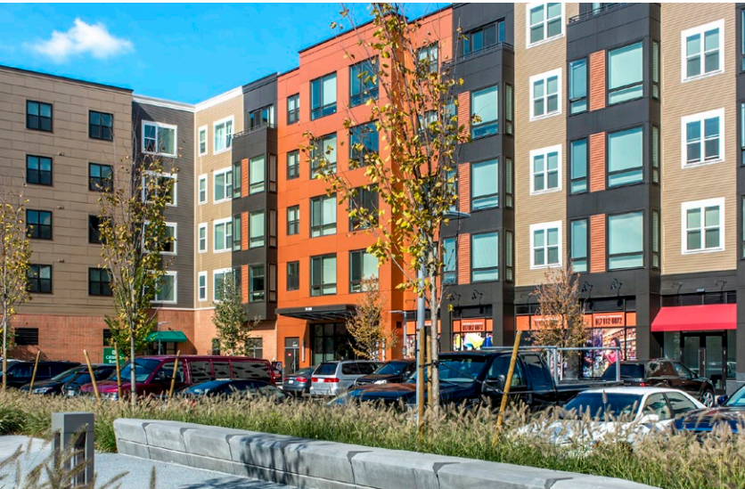
UPGRADE+TRANSFORM This typical wood-frame structure is articulated to appear as many buildings.
