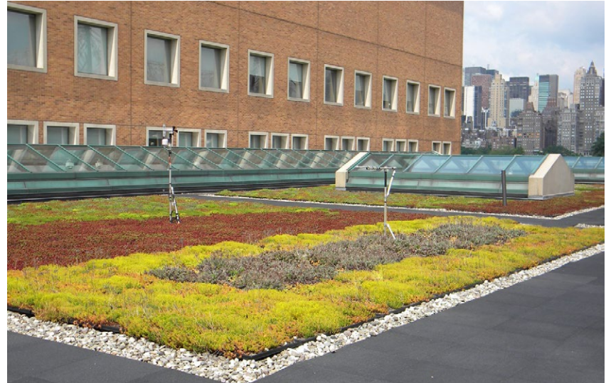
UPGRADE+TRANSFORM Horizontal roofs are recommended to include green infrastructure for stormwater.
