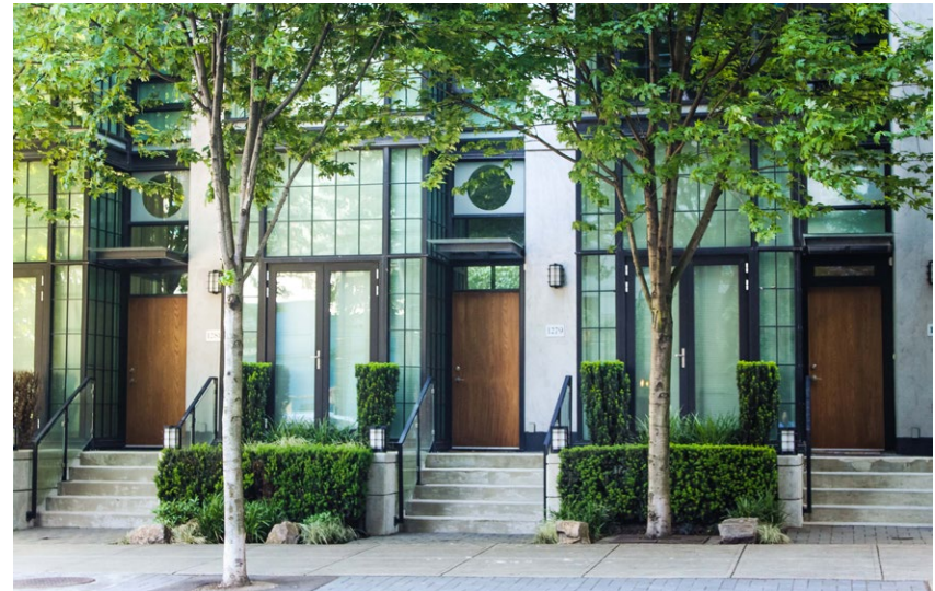
TRANSFORM Ground floor units are slightly elevated to provide privacy.
