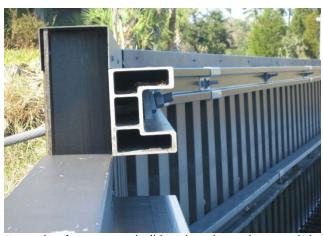
Example of composite bulkhead, wale, and cap with hot dipped anchor tie rods.
