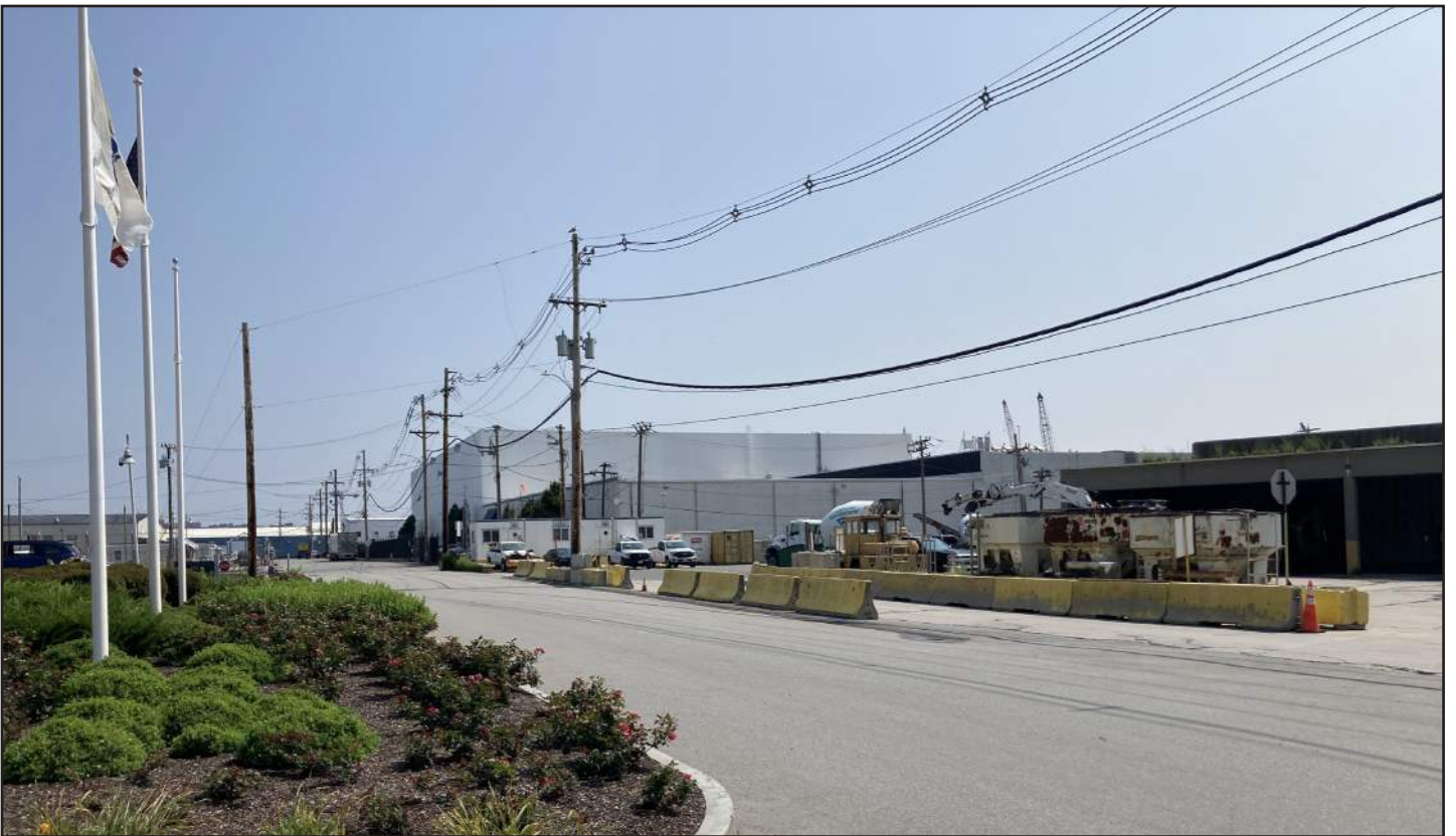
Photograph 16: View looking north from Constellation Energy towards Commercial Street
