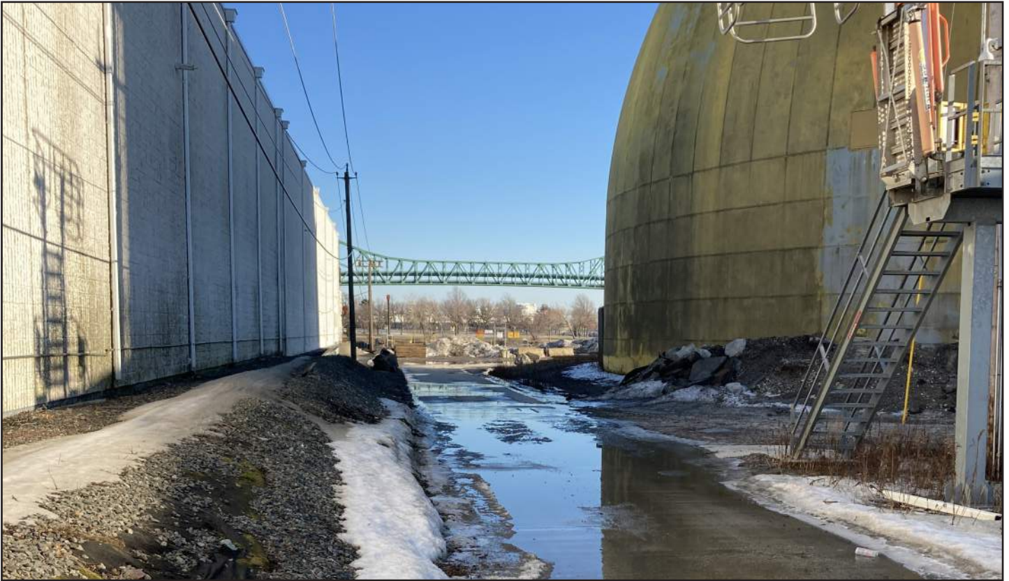
Photograph 13: View looking east towards Island End River, between Lineage Logistics and Quebec Cement
