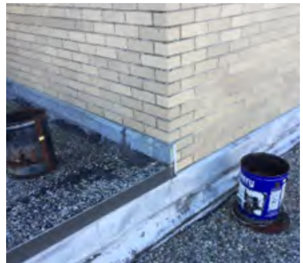
Flashing deteriorating
