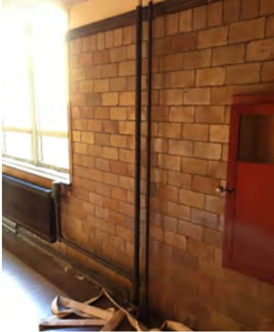
Glazed masonry wall
