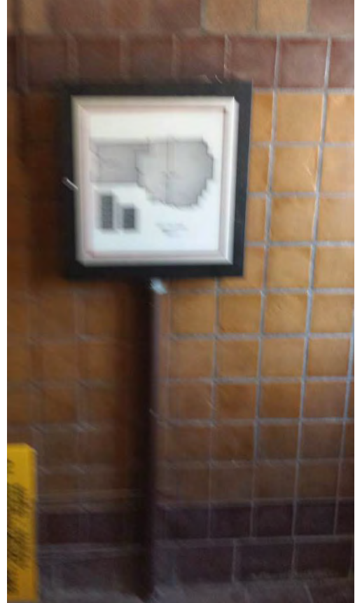
Annunciator in Man Entrance Lobby
