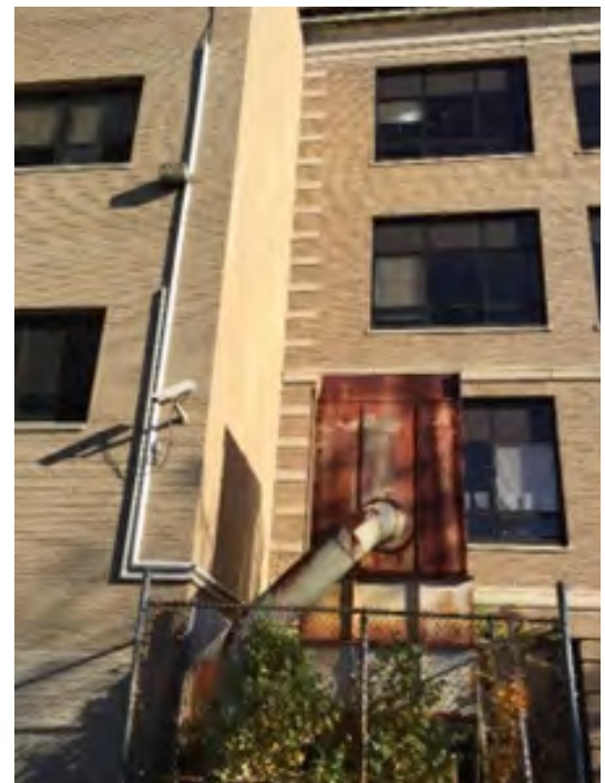
1970's addition and 1920's original building connection
