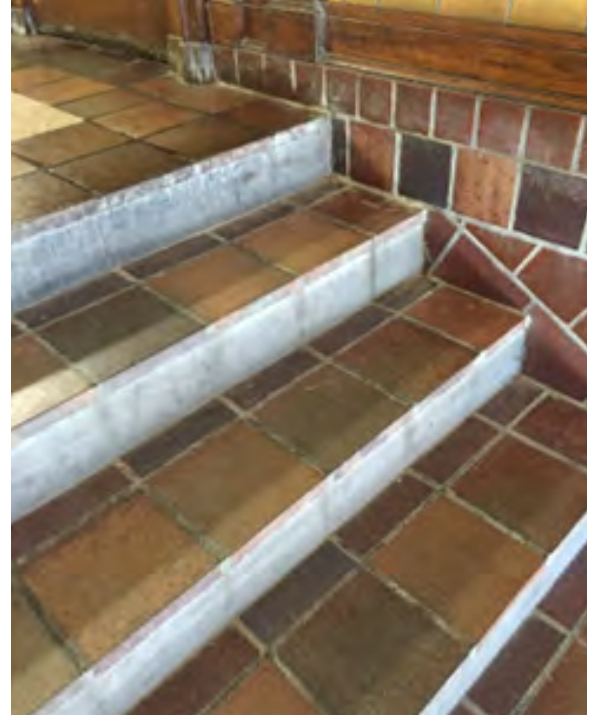
Tile stair treads main entry stair
