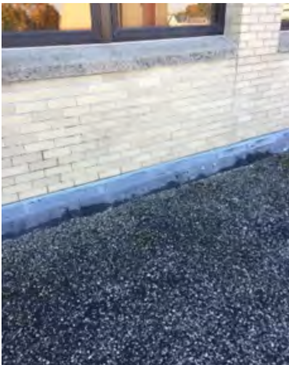
Tar and gravel roof, continuous thru-wall flashing
