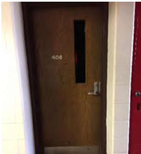
Original wood door system with hardware upgrade
