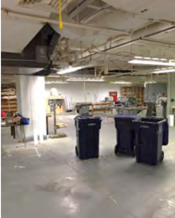
Painted concrete floors in shops
