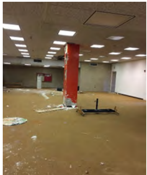
Existing Library space, acoustic tile, carpeted floor
