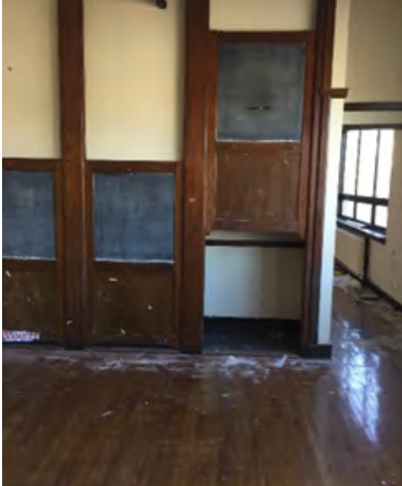
Wood flooring in classrooms
