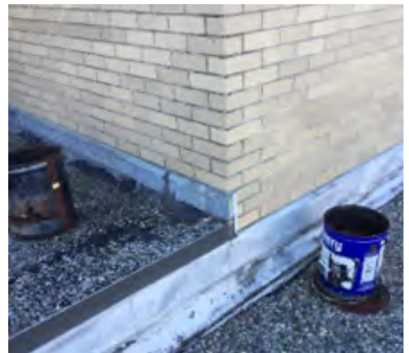
Flashing deteriorating
