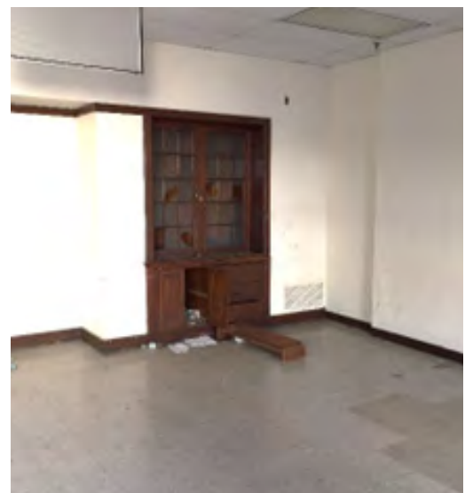
Classroom with painted plaster
