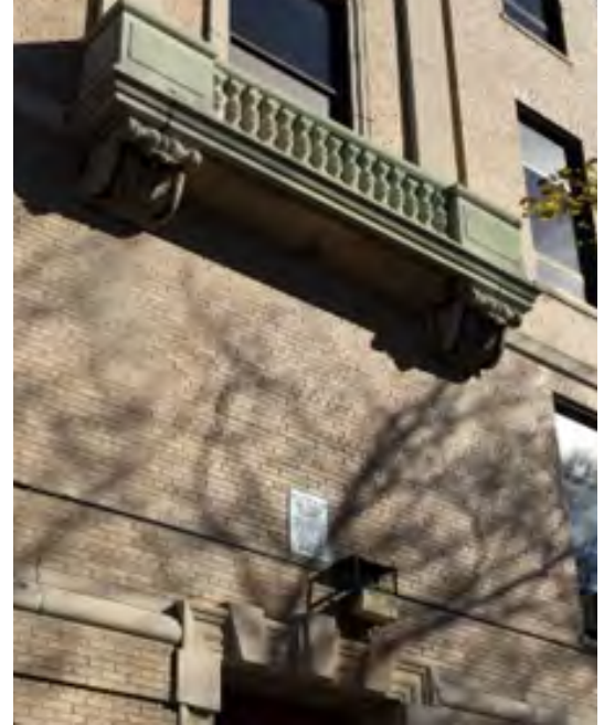
Ornamental cast stone balconies
