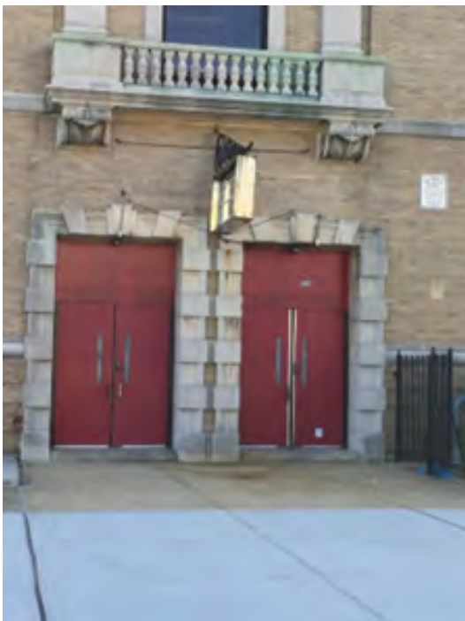
Ornamental cast stone, metal doors & frames
