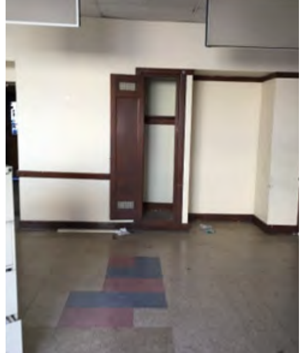
VCT & VAT floor in classroom
