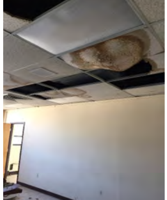
Classroom acoustical ceiling tiles
