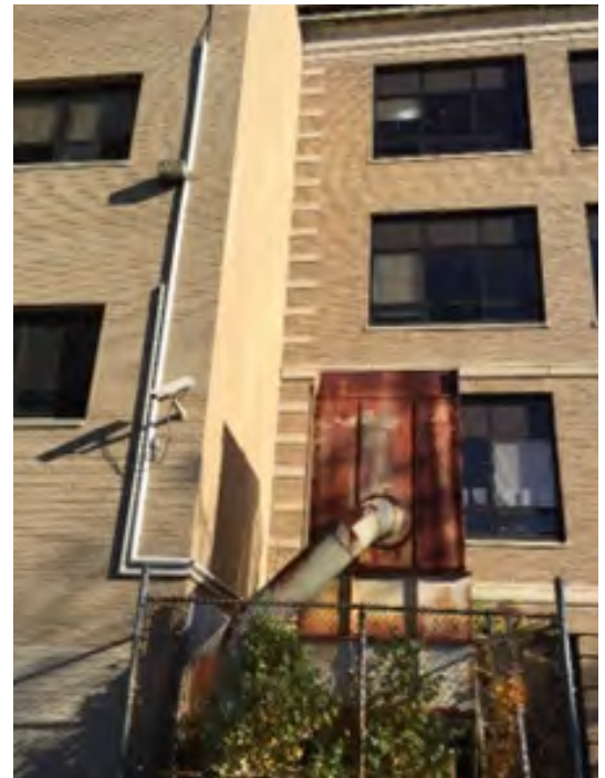
1970's addition and 1920's original building connection
