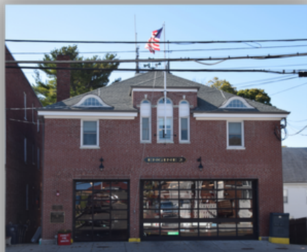
Hancock Street Station 54 Hancock Steet
