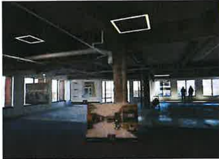
An office building near South Station is being converted to lab space, but the project is nearly complete and only about one-fifth of its square footage has been leased. It is one of a huge swath of projects that are coming online around Greater Boston, many of which are in their square-foot, 30,000- to 400,000-sq-ft range.
