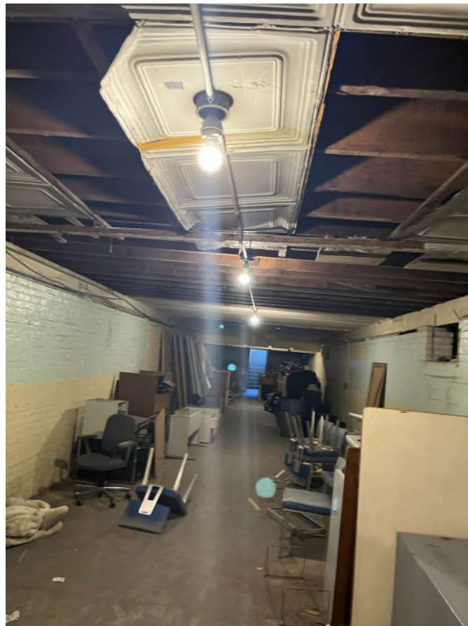
Figure 9: Unconditioned basement area with opening to conditioned first floor area
