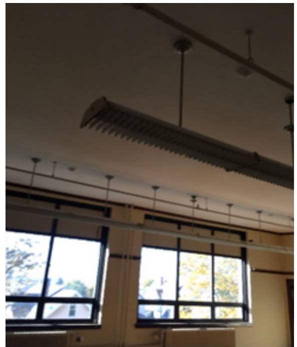
Classroom plaster ceilings
