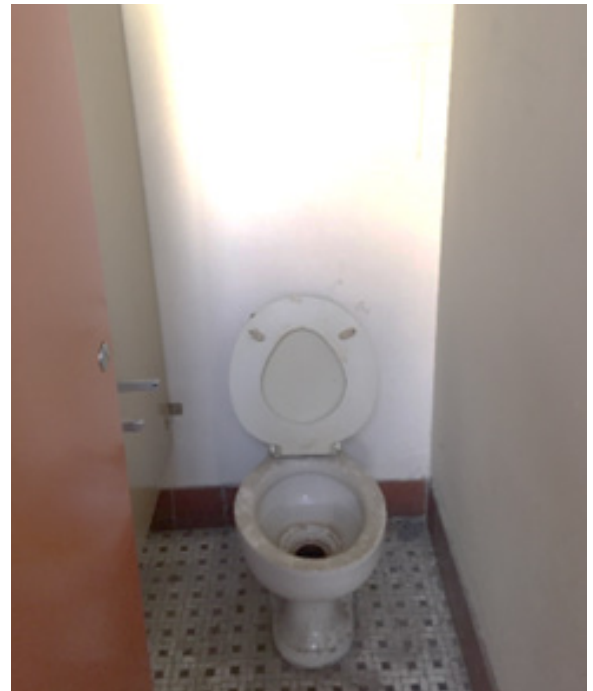
Ceramic tile in toilet rooms
