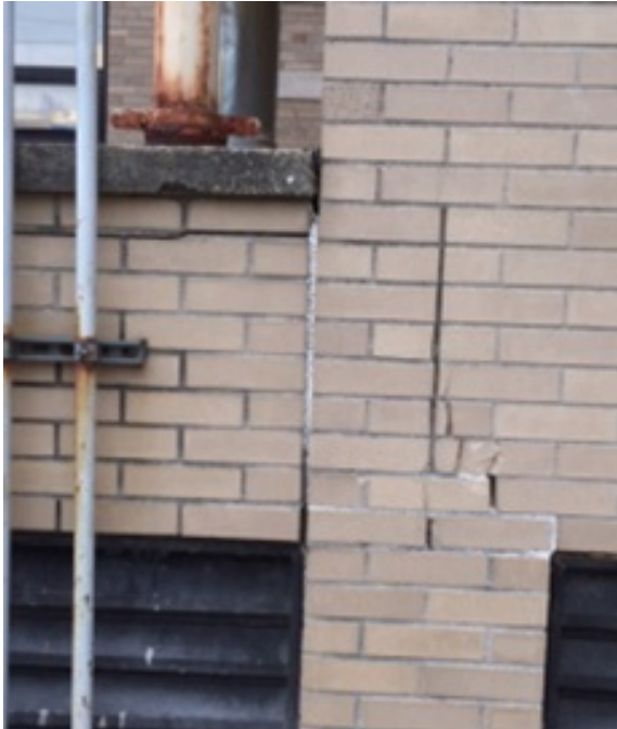
Some of the existing steel lintels were observed to be moderately rusted over window openings and the mortar joints at the ends of the loose steel lintels have spalled and show signs of gaps.
