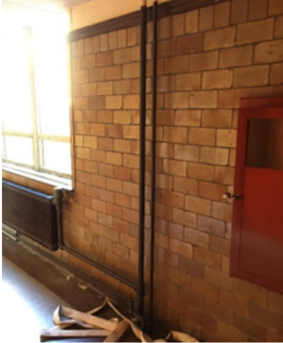
Glazed masonry wall
