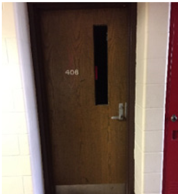
Original wood door system with hardware upgrade
