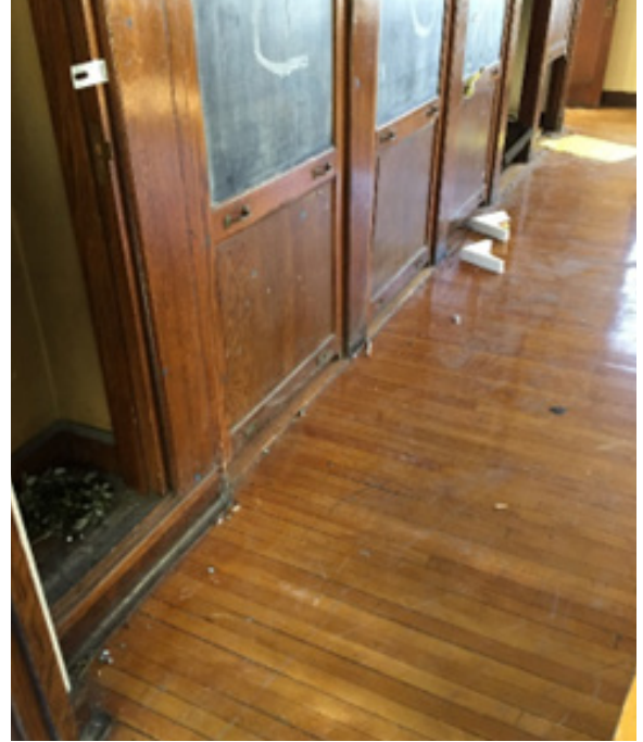
Existing wood floors typical in 1920's building classrooms
