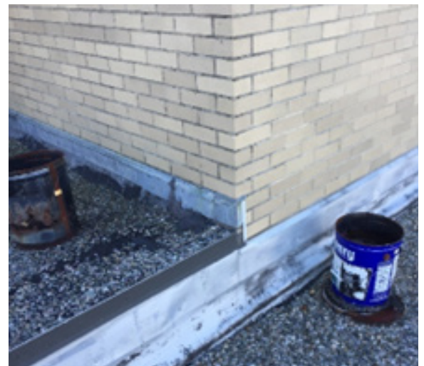
Flashing deteriorating
