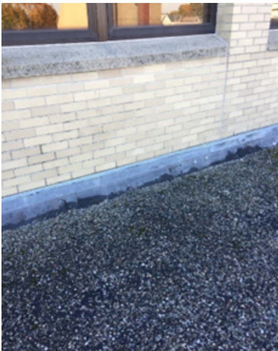
Tar and gravel roof, continuous thru-wall flashing
