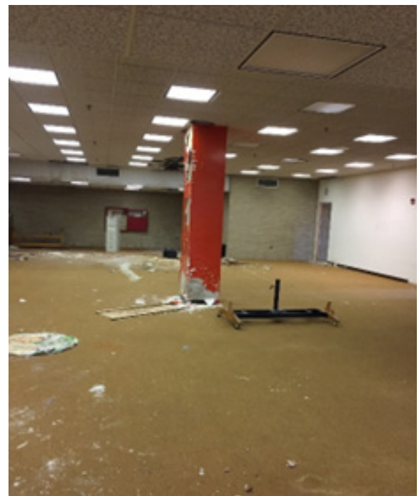
Existing Library space, acoustic tile, carpeted floor
