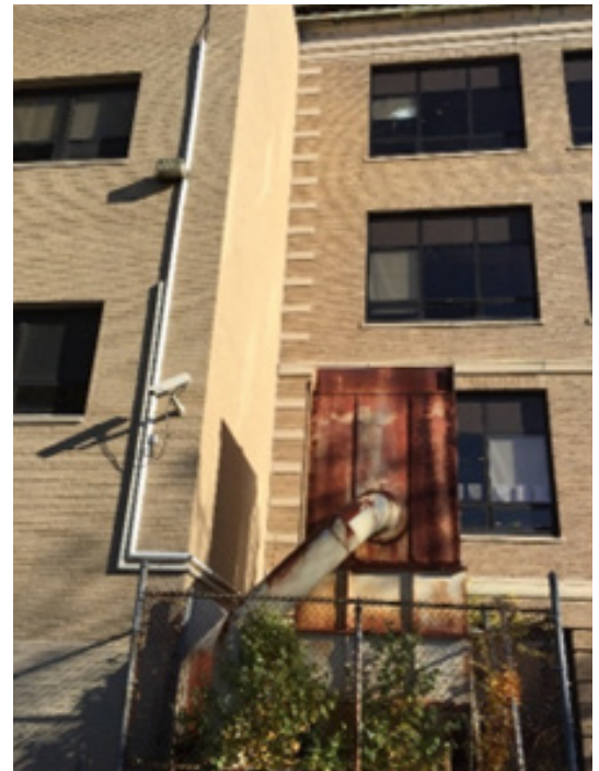
1970's addition and 1920's original building connection
