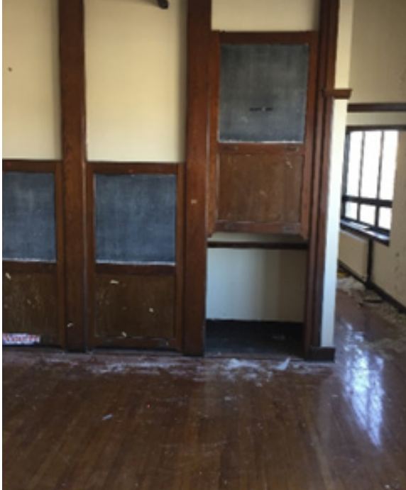
Wood flooring in classrooms
