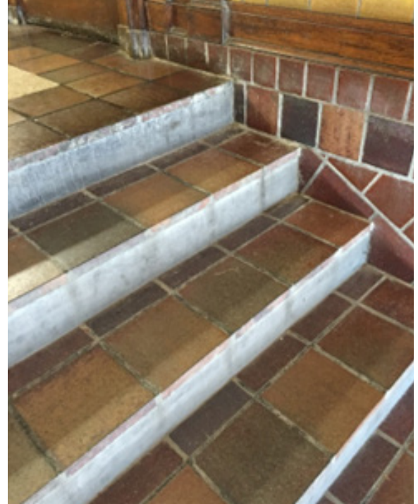
Tile stair treads main entry stair
