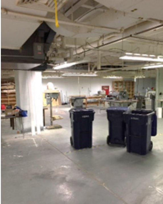
Painted concrete floors in shops
