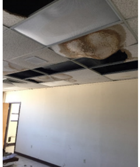
Classroom acoustical ceiling tiles
