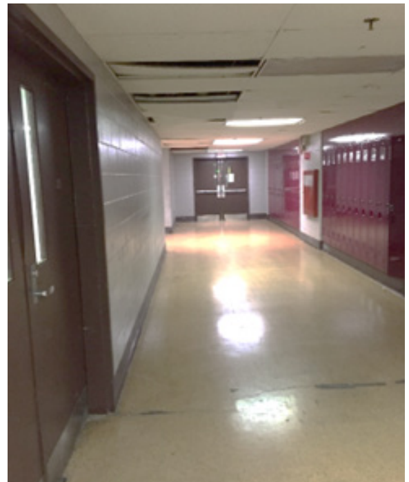
Existing VAT flooring materials
