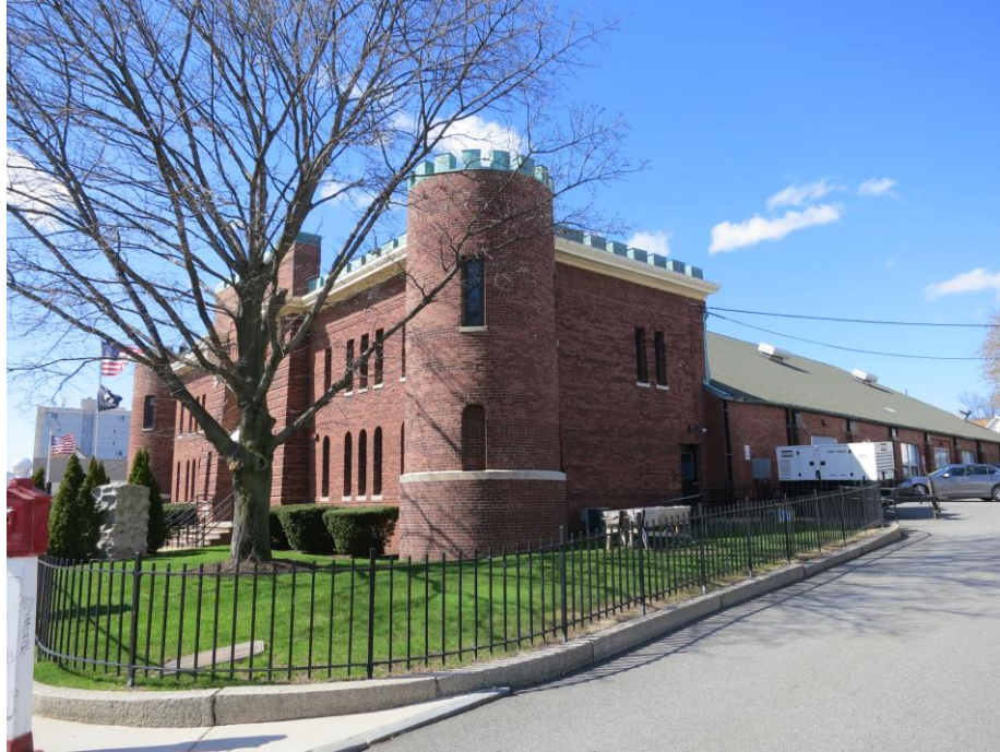
Photo 2 – view looking NW with former drill shed to rear
