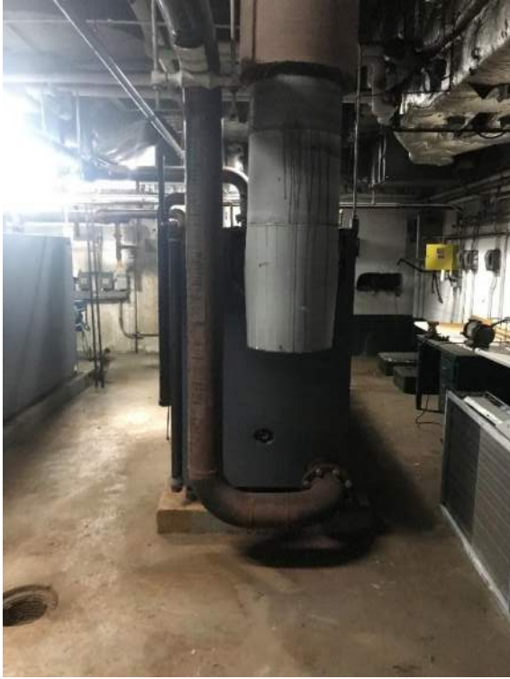
Concrete floors in Mechanical spaces
