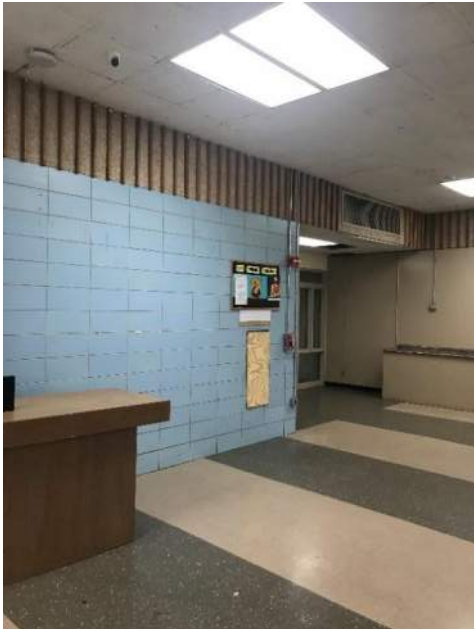
Stack bond block and acoustical treatment Meeting room
