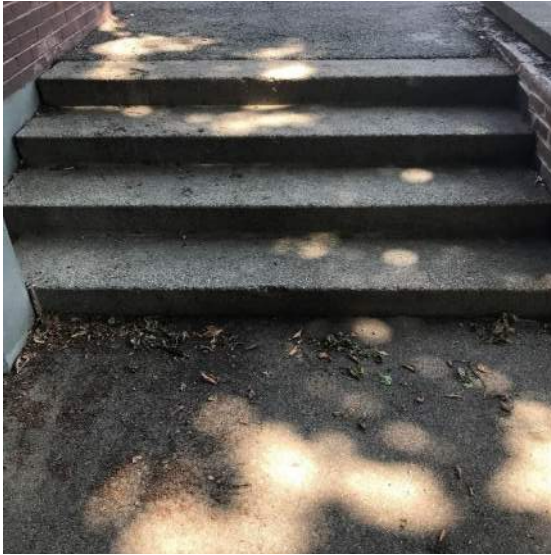
Concrete site stair/Accessibility
