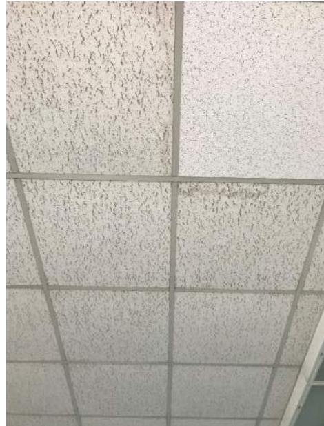
Typical ceiling tiles
