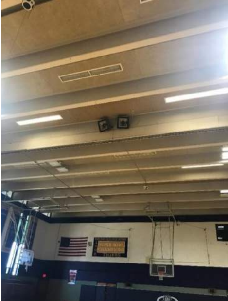
Exposed concrete beam and panel Ceiling between
