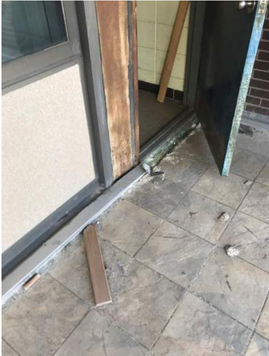
Stone pavers at exterior covered area
