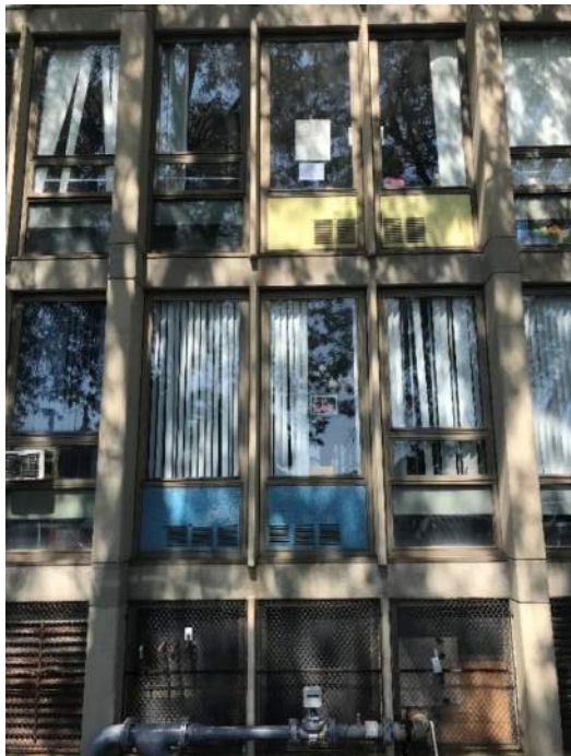
Original metal frame, porcelain panel and single pane glazed curtainwall system
