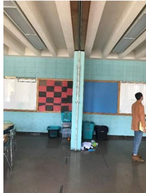
Painted stack bond in classroom
