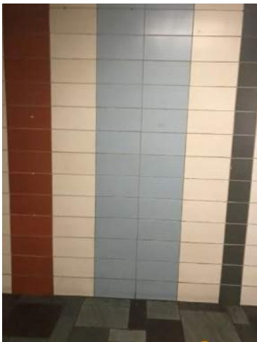
Stack bond structural glazed block
