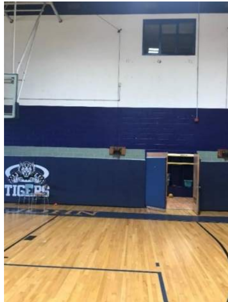
Painted stack bond concrete block in gymnasium
