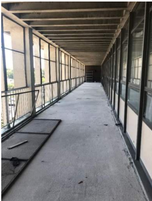
Exposed structure at covered area
