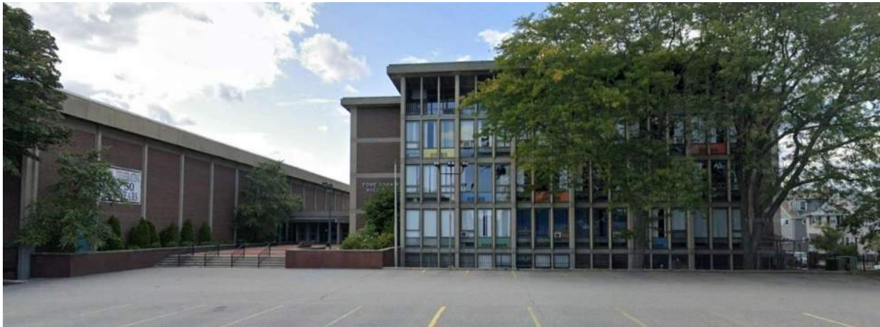
East elevation at main parking lot
