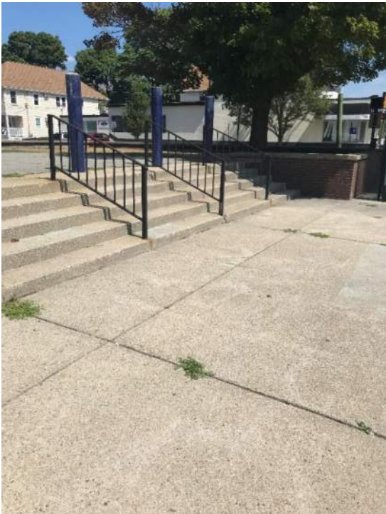
Concrete site stair Broadway/ Accessibility
