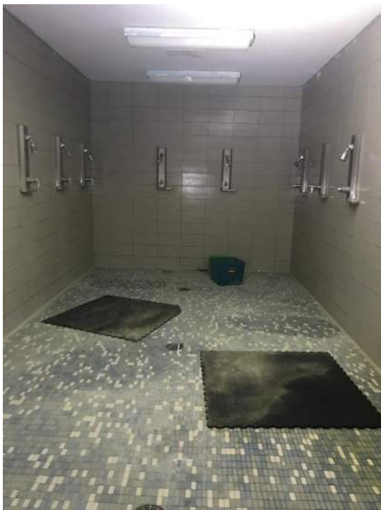
Existing boys gang showers. No longer used Not handicap accessible
