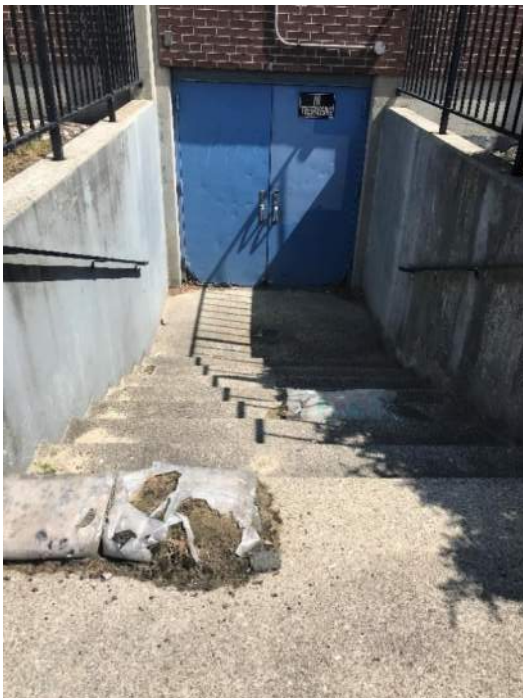
Exterior stairs to stair well
