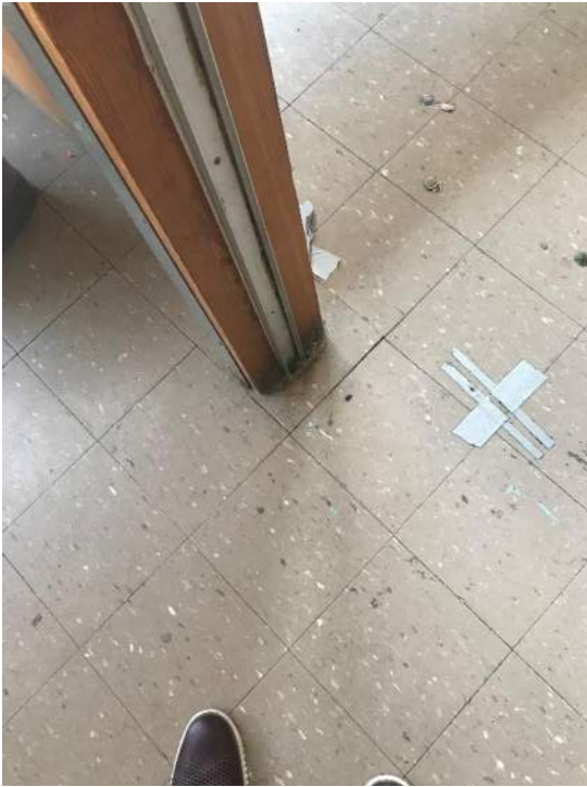
VAT flooring typical
