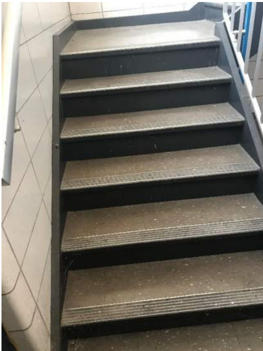
VAT at stair w/ nosing
