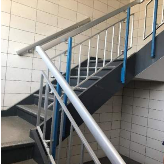
Aluminum handrails and ballasts
