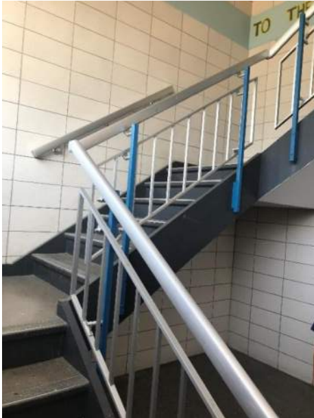
Stack bond glazed block in stairwell
