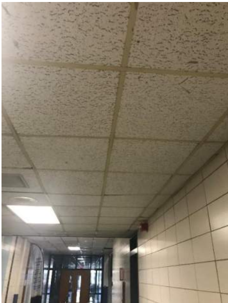
2 x 4 ceiling tile in corridor area
