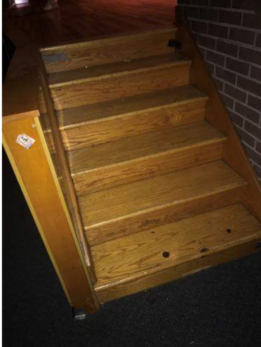
Wood stairs and risers at stage
