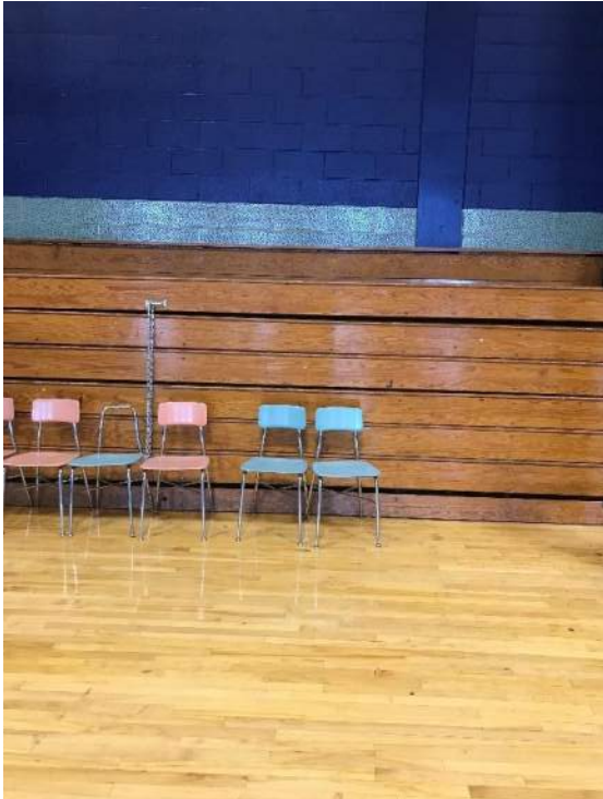
Wood gym floor, and original bleachers
