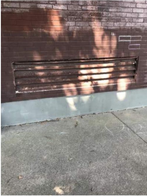
Mechanical louver in brick masonry
