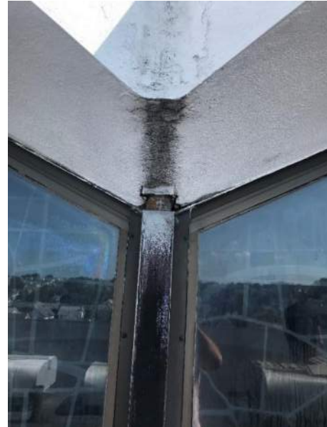
Corner downspout between windows
