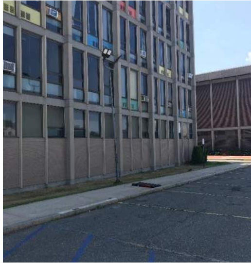
West elevation at rear of building/additional parking
