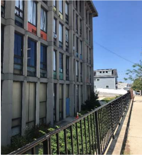
North elevation along Cameron Street
