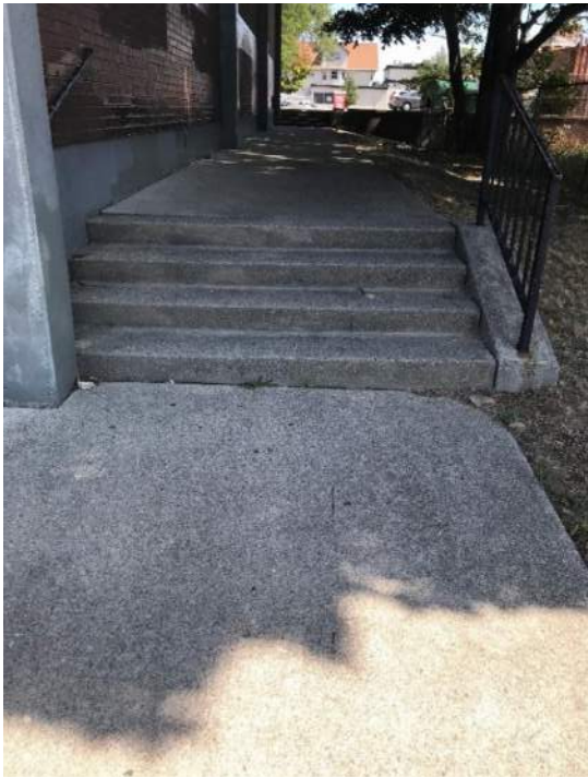
Concrete site stair and rail
