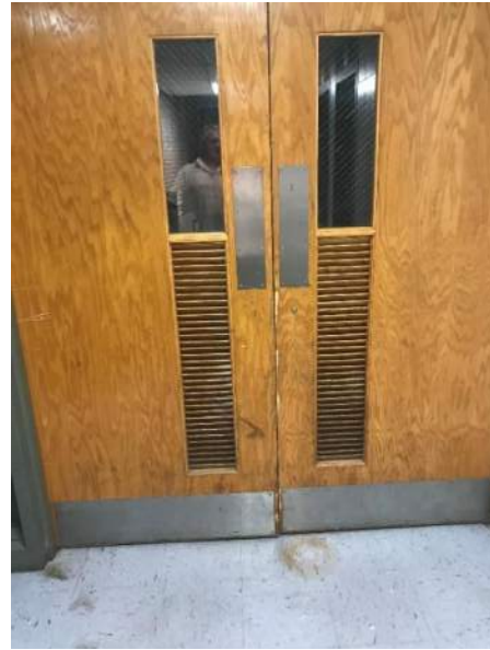
Glazed and louvered door
