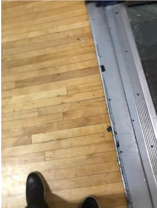
Original Wood Gym floor and aluminum sill
