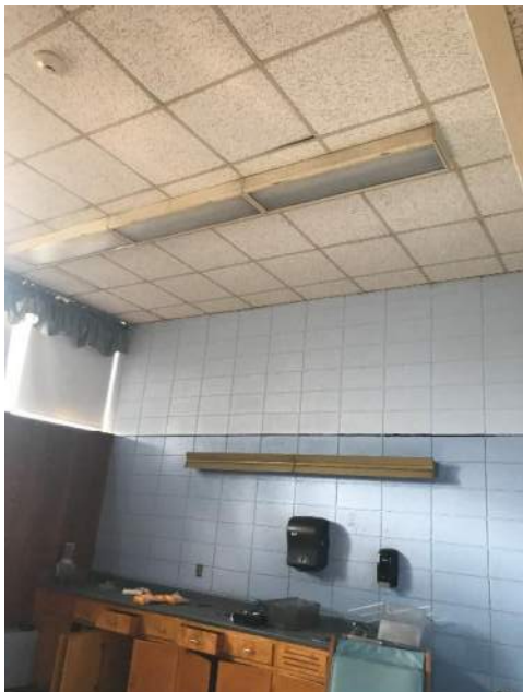
Stack bond in Classroom
