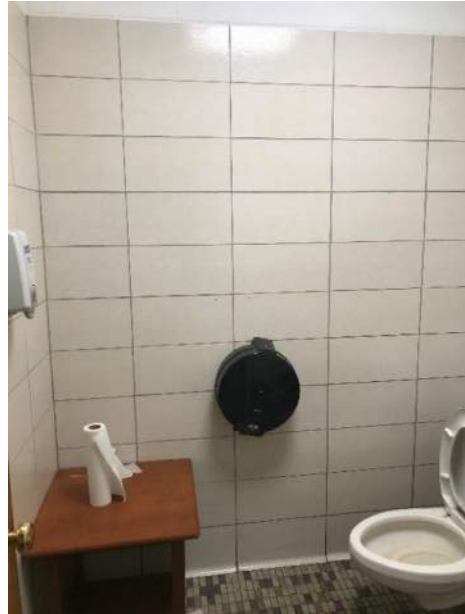
Stack bond glazed block @ toilet
