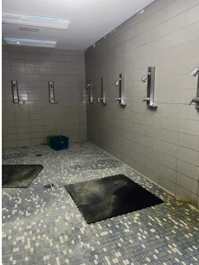
Boys Shower with central drains
