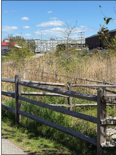
To reduce flooding and reconnect the stormwater system in the Air Force Road area to the Malden River, construction debris was removed and invasive plants removed to restore a naturalized streambed to South Creek. It is part of the City's overall plan. Native plantings and a wildflower mix were added to revegetate the area. Phase II will begin in 2026.
